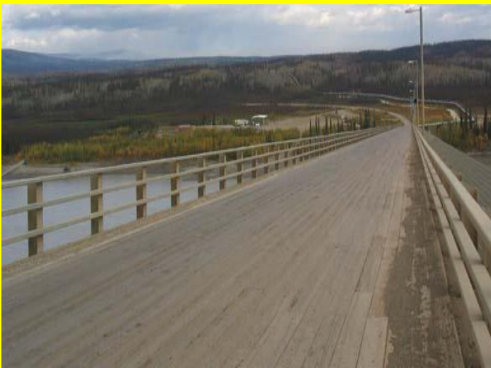
The Yukon River Bridge
