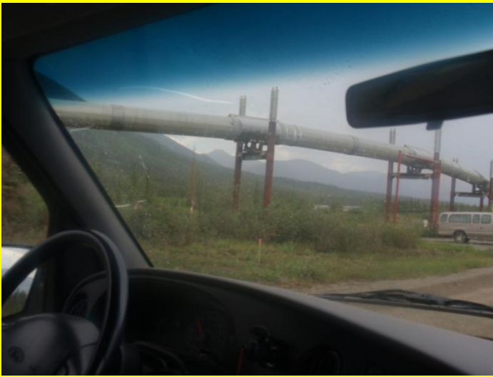
The pipeline runs along the highway.
