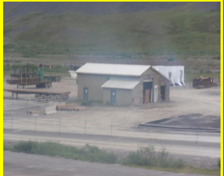
Pipeline Pump Station 3
